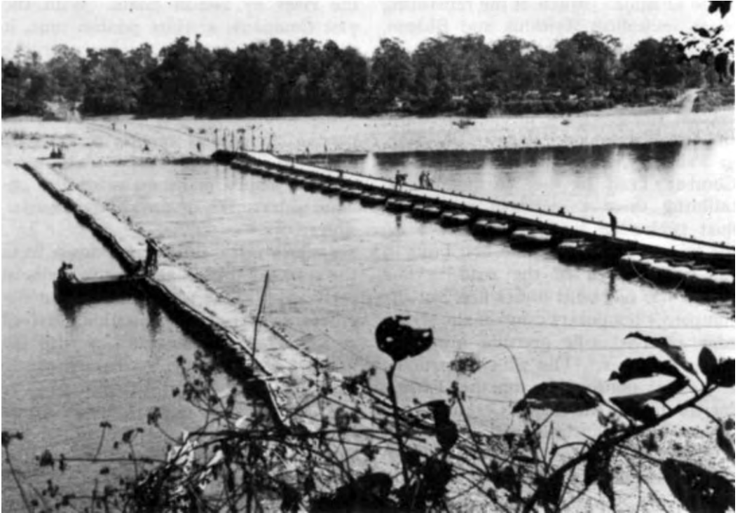
12-TON PNEUMATIC FLOAT BRIDGE BUILT OVER THE TARUNG RIVER, BURMA
